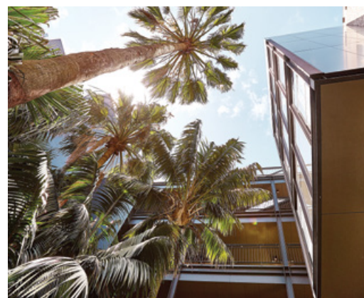
17 DANKS STREET, WATERLOO. BUILT BY MADE PROPERTY.
