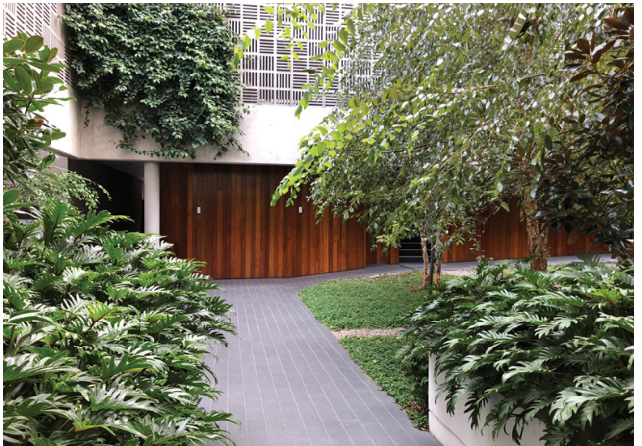
17 DANKS STREET, WATERLOO. BUILT BY MADE PROPERTY.
