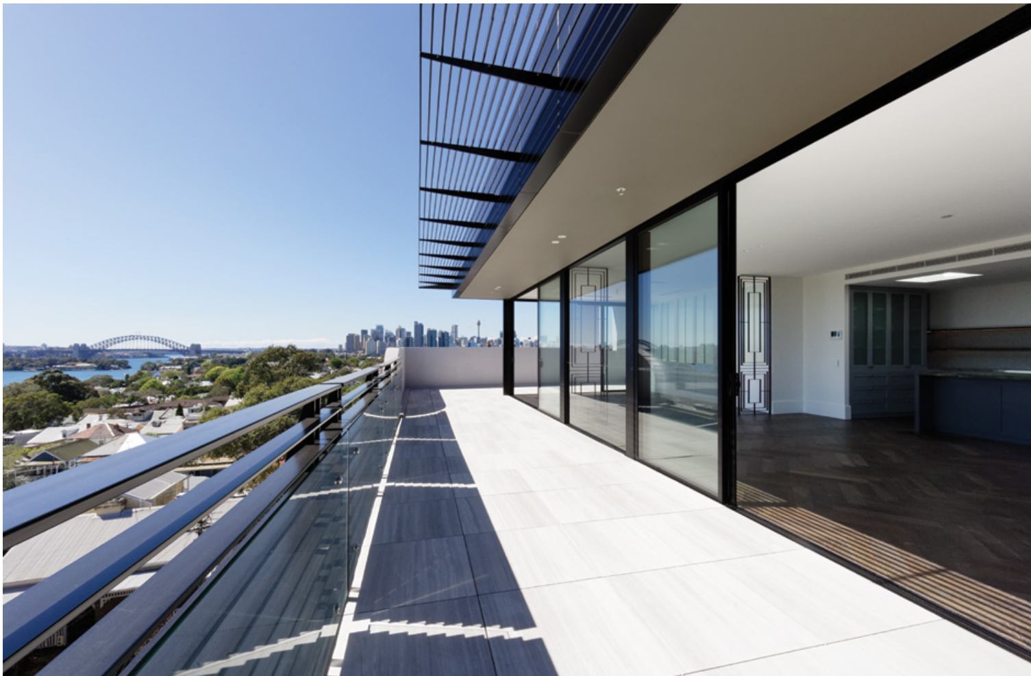
2A ROWNTREE STREET, BALMAIN. BUILT BY MADE PROPERTY.
